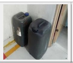
NC Photo 02: Machine oil drum without secondary containment
